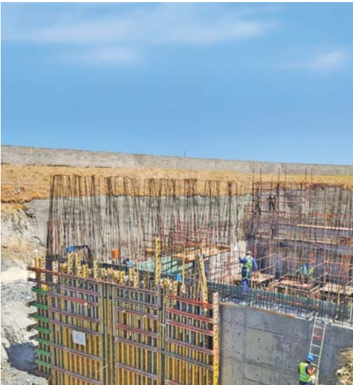
Building sanitation capacity: The Trappies bulk sewer rehab and Gordon's Bay pump station construction are key infrastructure upgrades that will help tackle sewer overflows in Strand and Gordon's Bay. The first to be delivered will be the Gordon's Bay pump station project, with construction over halfway (pictured top left) and about a third of the rising main installed (top right).
