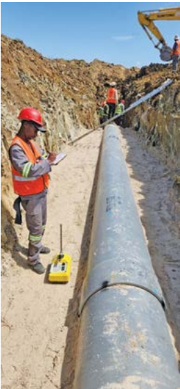
Building sanitation capacity: The Trappies bulk sewer rehab and Gordon's Bay pump station construction are key infrastructure upgrades that will help tackle sewer overflows in Strand and Gordon's Bay. The first to be delivered will be the Gordon's Bay pump station project, with construction over halfway (pictured top left) and about a third of the rising main installed (top right).
