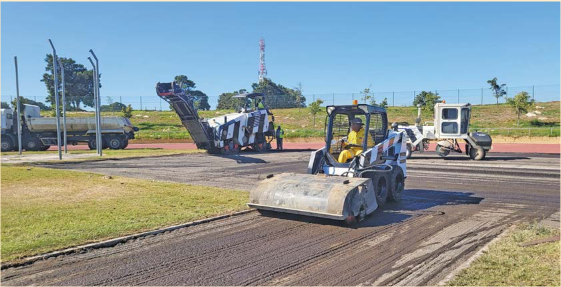
On the winning track: The phased refurbishment of the Blue Downs athletics track is progressing well. The upgrade includes resurfacing, and improving key features such as the hammer throw cage, take-off boards and steeplechase area.
